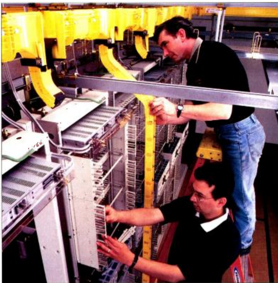
While installing fiber cable, strict adherence to guidelines regarding its flexibility must be observed. Raceways, such as those being installed here, help to organize and protect cable, as well as ensure the integrity of its location and minimum bend radius over time. Photo courtesy ADC Communications.
